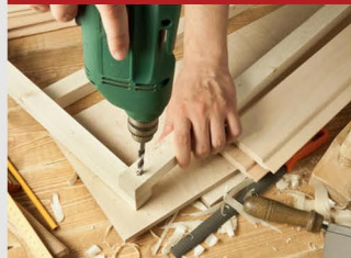
General Carpentry Repair
